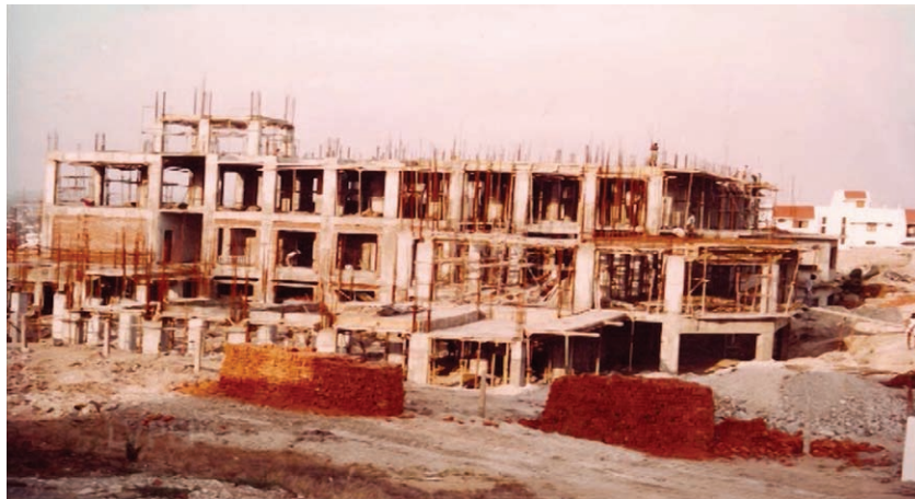
Building construction in six months.
